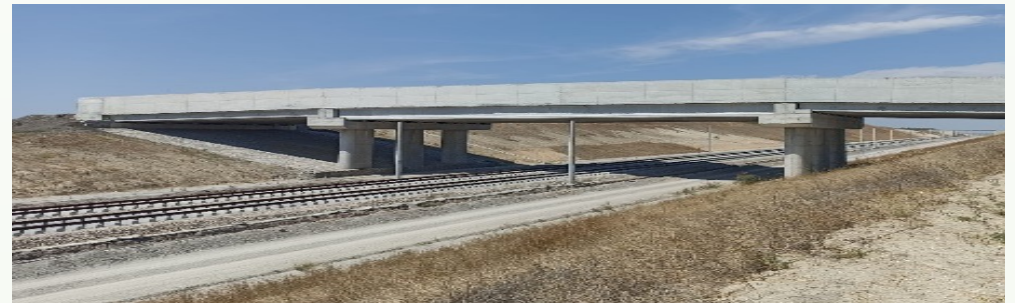
Photograph 2. Wildlife Crossing Bridge
